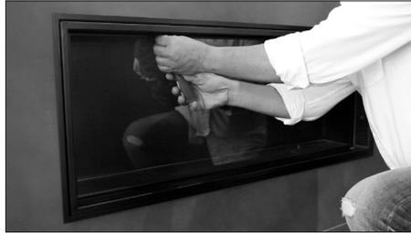
**Step 3:** Pull the upper tabs and tilt the glass towards you. Then carefully lift and detach from the bottom two pins.
